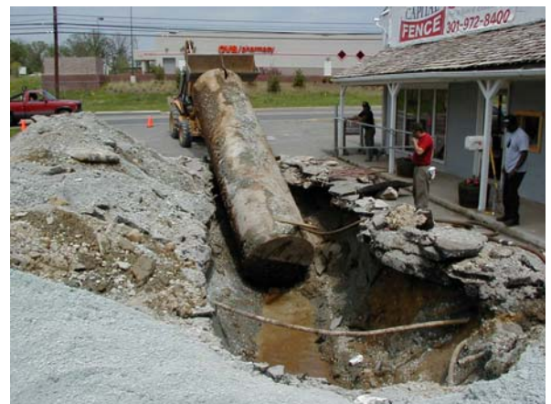
Removal of a 4,000-gallon underground fuel storage tank.
