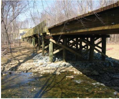
Timber pilings and cross-bracing.
