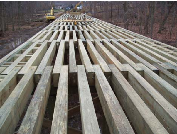
Timber and asphalt bridge construction.
